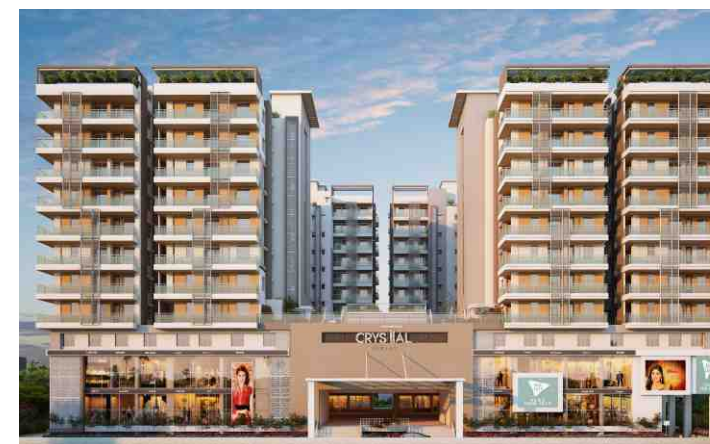
CRYSTAL TOWERS Danapur – Khagaul Road, Patna
